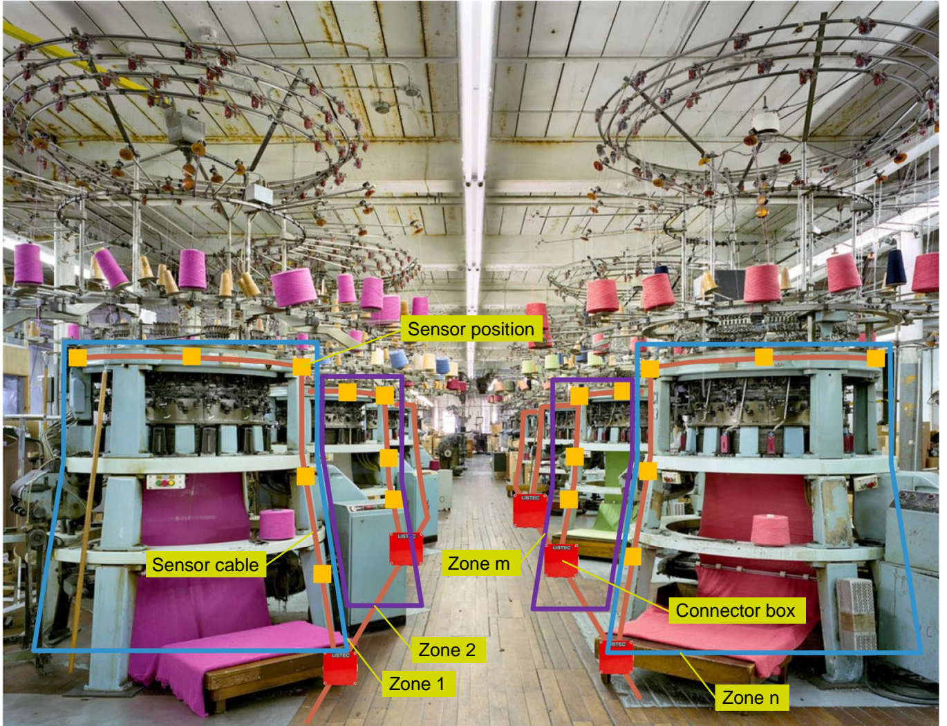
(b) SecuriHeat d-LIST sensing cable layout design as one alarm zone per machine
