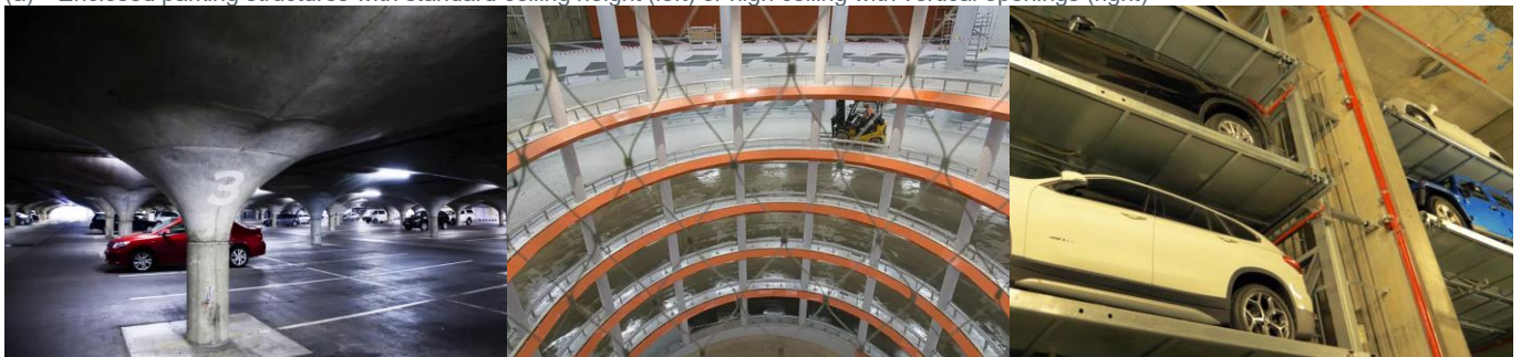
(b) Carparks with irregular roof structure (left) or through innovative design (e.g. cylindrical carpark or automated car stackers (right))
