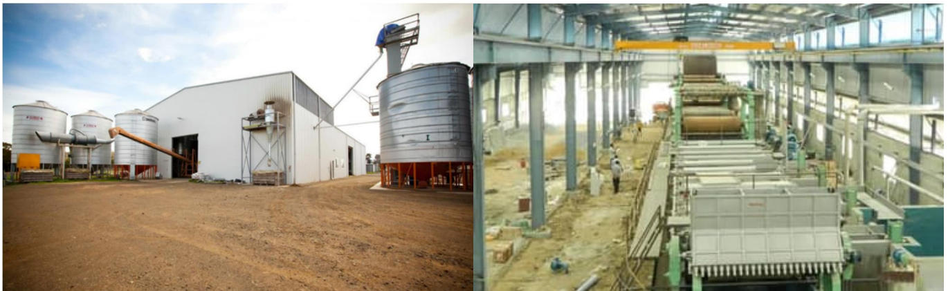
(a) Examples of partially enclosed manufacturing areas (left: food processing; right: paper mill)
