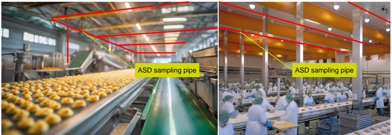
(a) ASD pipe layout at ceiling level with exposed roof structure or flat with voided ceiling
